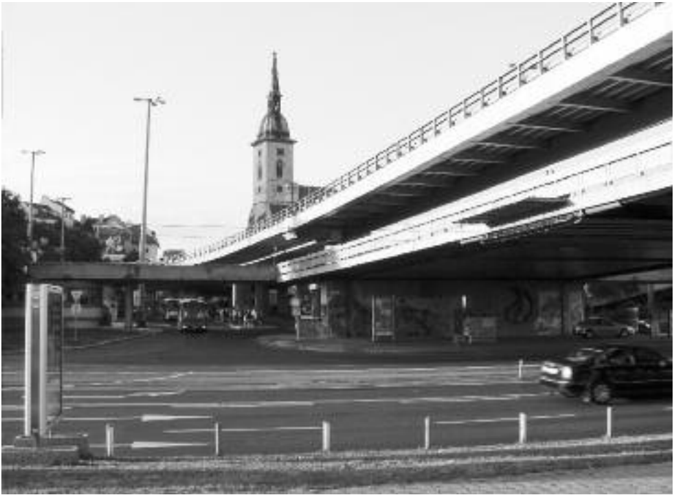
The bridge and the road at the demolished Podhradie zone. Photo: D. Luther, author's archive.
